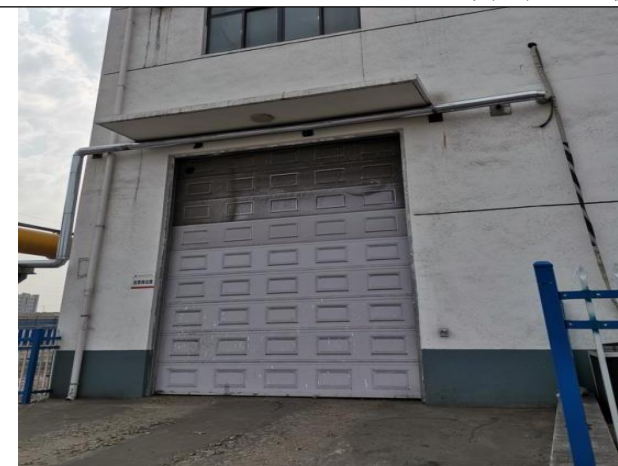
脱硫石膏暂存库
