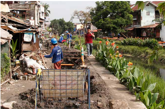
⌵ During construction of sewerage network
